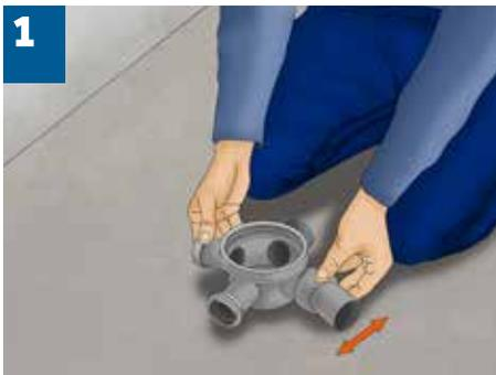
**1** Selection of the appropriate base and the corresponding drain assembly. Installation of a selected base with a ball (output Ø 50) on the bathroom floor in proper position for connecting of other cables. Adjusting of output drain according to the situation in the bathroom.
