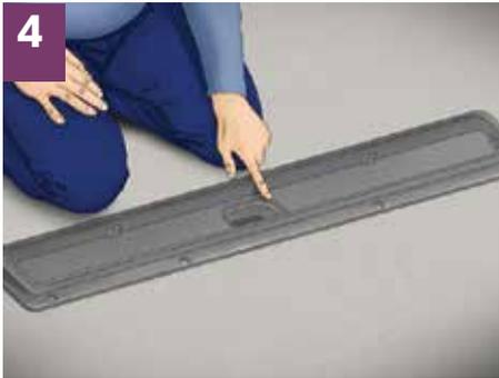
After setting a grate holder and its adjustment, leveling layer on the bathroom floor is made, up to the level of grate holder.
