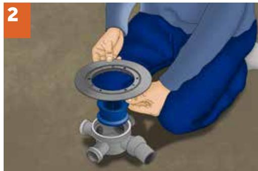
**2** During installation make sure that all rubber seals are lubricated. Insert a socket in the base. Setting of a hoop for hydro isolation to the selected base. Setting up of layers of flat roof.
