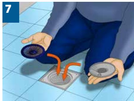
**7** Inserting of a grid for hair (or irreversible valve - depending on the customer's choice)
