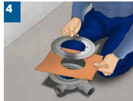
**4** Installation of flange for hydro isolation. Between it and hoop, hydro isolation is inserted. It is tightened with screws so that hydro isolation cannot fall out (pull through).
