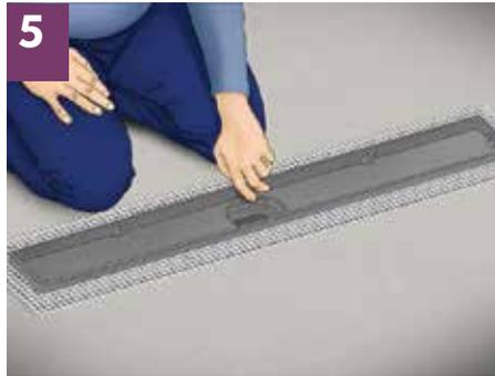
Then, setting up the reinforcement mash for the hydroinsulating layers and its connections with selected insulating materials in the bathroom.
