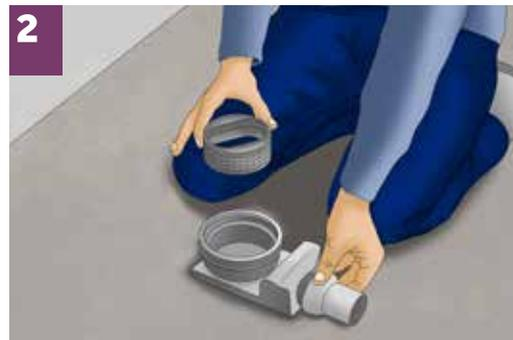
**2** During installation make sure that all rubber seals are lubricated. Before the holder of a grate, reducer for linear drain is set, on which grate holder of linear drain is placed.
