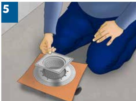
**5** Inserting - setting of grid carrier and its adjusting according to the height and slope.
