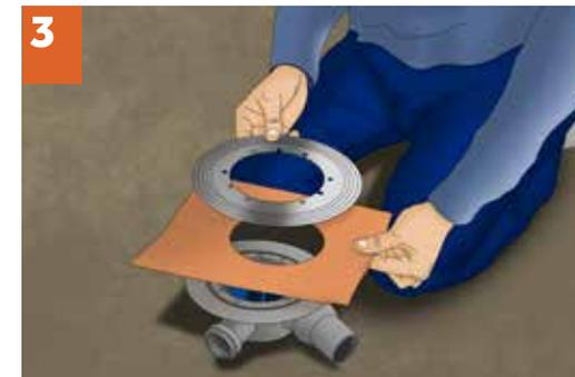
**3** Installation of flange for hydro isolation. Between it and hoop, hydro isolation is inserted.
