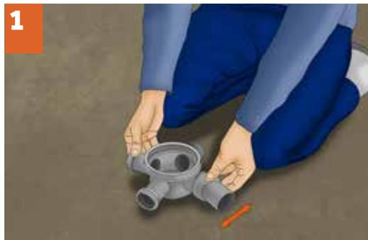
**1** The first step of installation is choosing the proper base and corresponding drain assembly. Installation of a selected base with a ball (output Ø50) on the top in proper position for connecting of other cables. Adjusting the angle of output (exit) according to the situation.
