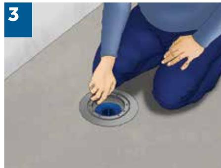
**3** After setting of a hoop for hydro isolation, leveling layer on the bathroom floor is made, up to the level of hoop.
