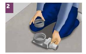
During installation make sure that all rubber seals are lubricated. Before the holder of a grate, reducer for linear drain is set, on which grate holder of linear drain is placed.
