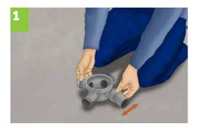
The first step of installation is choosing the proper base and corresponding drain assembly. Installation of a selected base with a ball (output Ø50) on the garage floor (driveway), or garden, in proper position for connecting of other cables.
