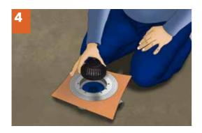
It is tightened with screws so that hydro isolation can not fall out (pull through). Setting of the final layer of flat roof, and then setting a grid for leaves.
