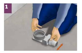
Setting of a base with the ball (output ø50) on the bathroom floor in the proper position. Adjusting the angle of a drain (output) according to the situation in the bathroom.
