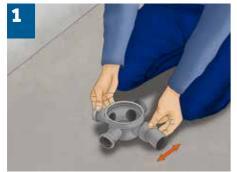
Selection of the appropriate base and the corresponding drain assembly. Installation of a selected base with a ball (output Ø 50) on the bathroom floor in proper position for connecting of other cables. Adjusting of output drain according to the situation in the bathroom.
