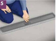
Then, setting up the reinforcement mash for the hydroinsulating layers and its connections with selected insulating materials in the bathroom.
