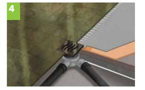
Setting the tiles or the chosen finish layer on the garage floor, driveway (if it is a grassed area, this step does not exist). Setting of a selected grid (stainless steel or cast-iron, depending on the wish of a customer).
