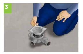
Inserting-setting of grid carrier and its adjusting according to the height and slope.
