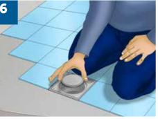
Inserting - setting of grid carrier and its Setting of a temporary safety cover. Setting of tiles on the bathroom floor.
