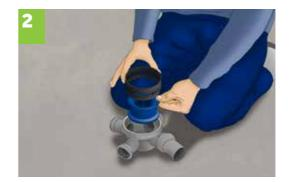
During installation make sure that all rubber seals are lubricated. Insert a socket in the base. Set up a grid for drainage.
