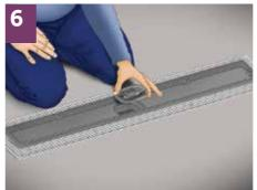
After setting up the hydroinsulation, hair stopper is inserted, and setting up the tiles in the bathroom can start.
