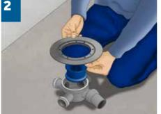
During installation make sure that all rubber seals are lubricated. Inserting of socket into the base (if we are talking about S base, this step does not exist, -S base does not have socket).
