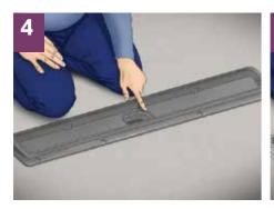
After setting a grate holder and it's adjustment, leveling layer on the bathroom floor is made, up to the level of grate holder.
