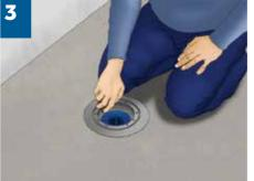
After setting of a hoop for hydro isolation, leveling layer on the bathroom floor is made, up to the level of hoop.
