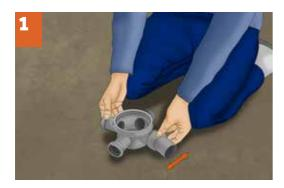
The first step of installation is choosing the proper base and corresponding drain assembly. Installation of a selected base with a ball (output Ø50) on the top in proper position for connecting of other cables. Adjusting the angle of output (exit) according to the situation.
