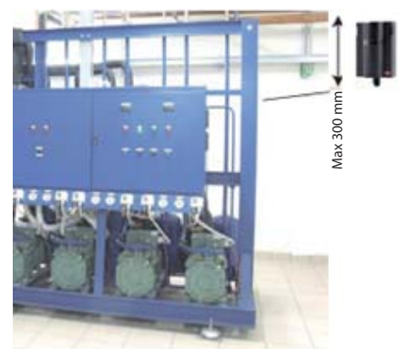
Per gas: NH 3 - ETHYLENE h max 300 mm from ceiling
