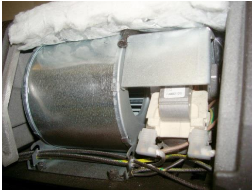
Figure No.9 - Access to fans
