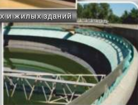
Baffle of equipment
