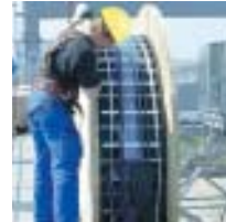
Top service – Assembly on site in a container facility.
